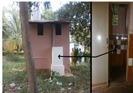
Fig no 5 Toilet, Government High School, arrow is shown to illustrate how the chute and incinerator are connected. Photo source: Author generated
